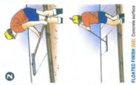
handle lowered, on the returns stroke the being levelled with a "buil float". On the forward stroke the float is pushed with float is pulled with the handle raised.
